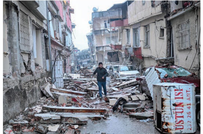
A man navigates the rubble in Hatay, Turkey, on Feb. 7. Rescue teams from around the world are pouring into the country and neighboring Syria after a pair of powerful earthquakes on Feb. 6 killed at least 12,000 and left millions homeless.
